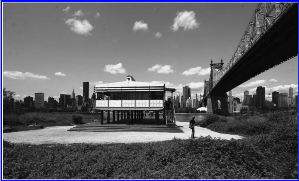
Jean Prouvé. Maison Tropicale. 1951. As installed on the waterfront in Queens, NY, May 2007. Photograph by Don Emmert/AFP/Getty Images.
